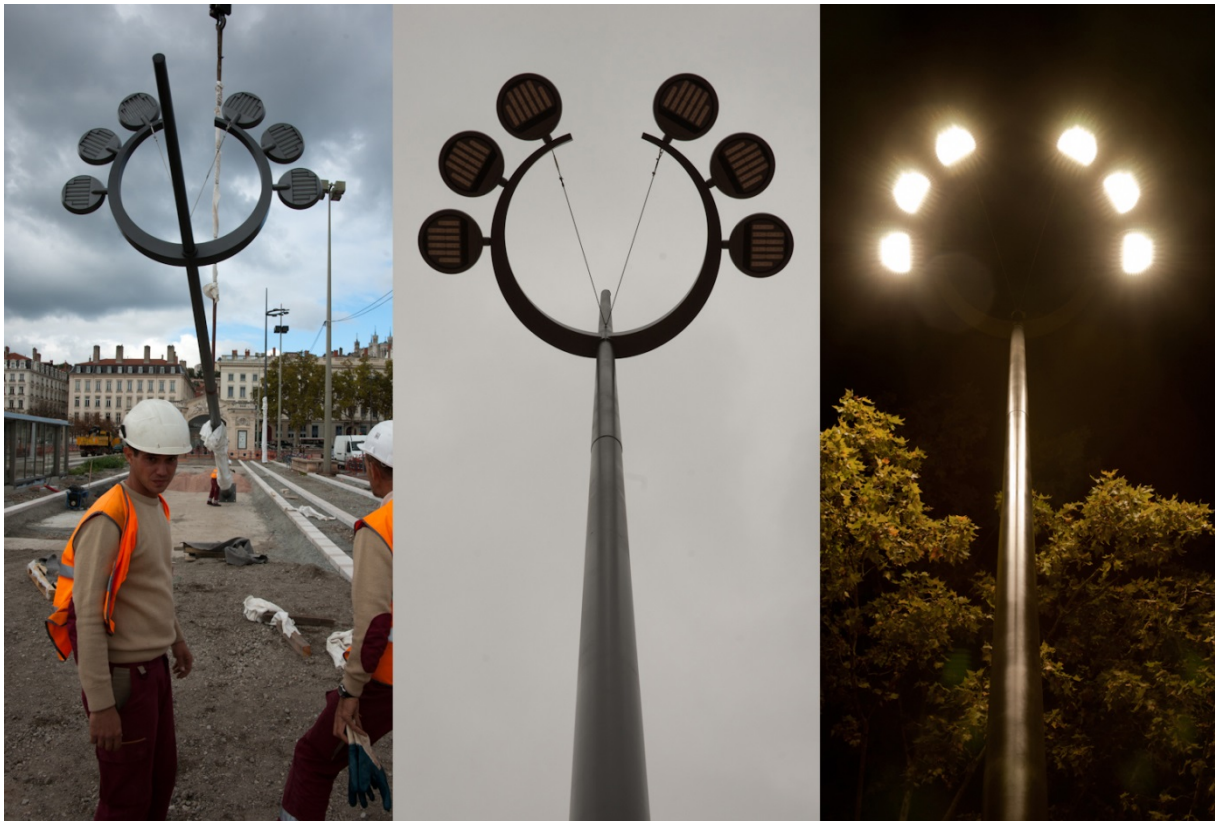
Figure 6-4: Crowns of six 120W LED luminaires heads at a height of 15 meters ©.
