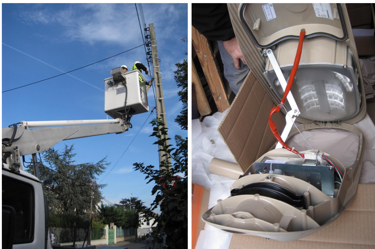
Figure 6-7: Routine installation works in Rue Thénard and an open new LED luminaire (CC).
